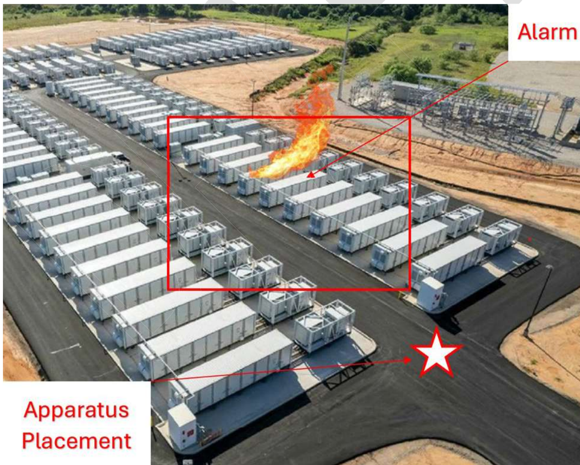
Figure 25 Safe Staging for Asset Protection
