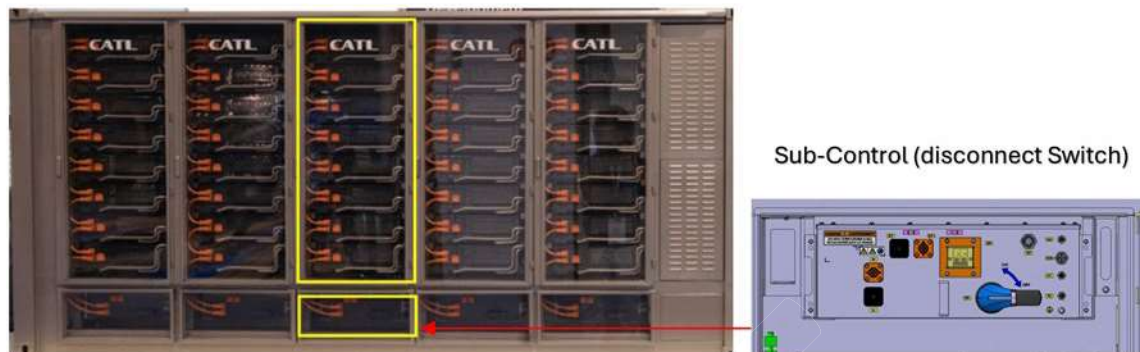
Figure 8 Battery String
